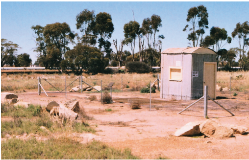
The Hines Hill weighbridge on 8 November 2008 with the former narrow gauge railway yard and the goldfields water pipeline behind.
